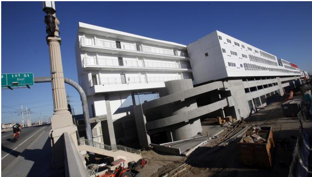
One Sante Fe in the L.A. arts district has 438 apartment units contained in a six-story-high, quarter-mile-wide structure. It const $165 million to build. (Bob Chamberlin / Los Angeles Times)
